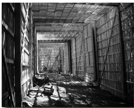
Completion of a 110 foot eagle flight cage
